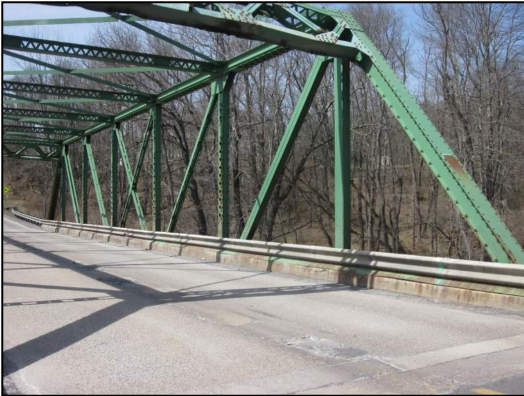
North/Downstream Truss, Roadway View, highlighting End Posts, Hip and Main Vertical Posts, and Diagonal Tension Members. View NW (WVDOH 4-5-2021)
