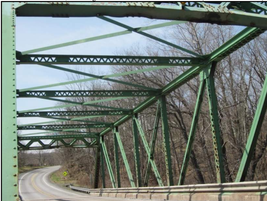
Highlighting Top of Bridge with Portal and Sway Stuts and crossed Lateral Bracing. View NW (WVDOH 4-5-2021)
