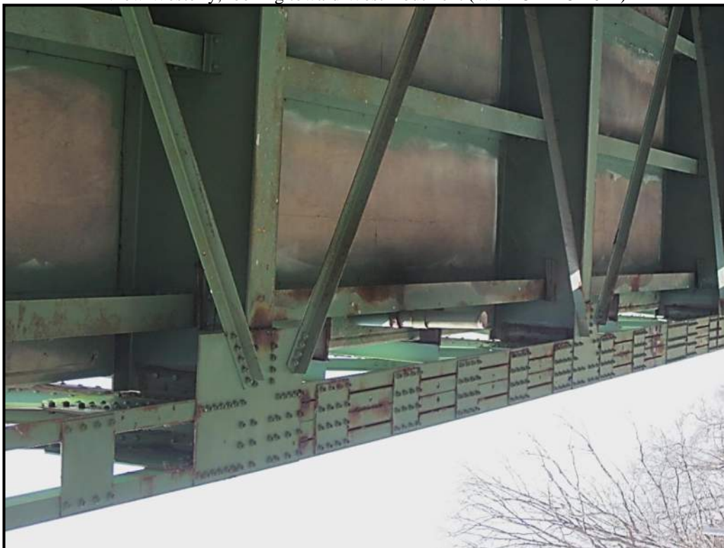
North/Downstream Truss, highlighting the Lower Chord arrangement, This image is rotated 90-deg counterclockwise. Note that this view mostly shows the mid-span of the lower chord with the four L-shape (angle) beam arrangement. The upper image shows a portion with the two L-shape arrangement. View Westerly, looking toward West Abutment (WVDOH 4-5-2021)
