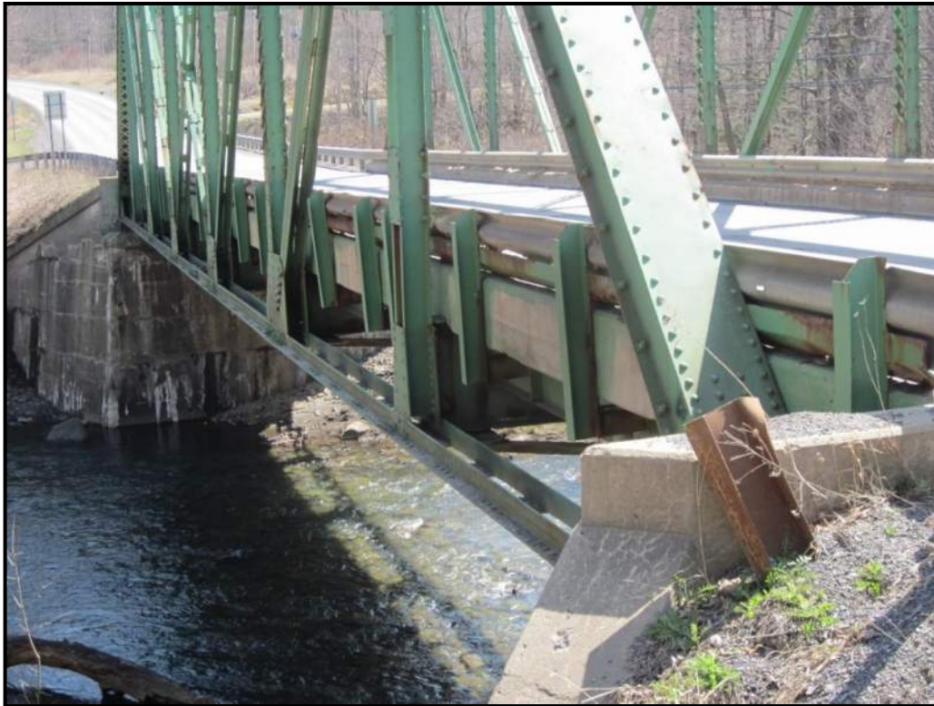
North/Downstream Truss, highlighting the Lower Chord arrangement. View Westerly, looking toward West Abutment (WVDOH 4-5-2021)
