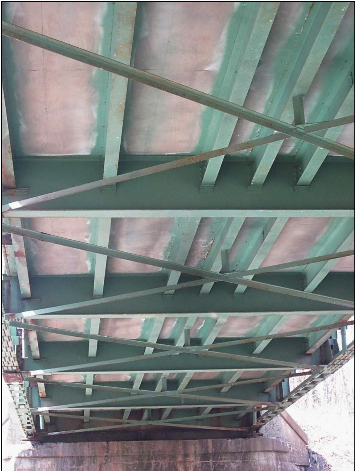
Underside of Superstructure, highlighting Floorbeams, Stringers and Lateral Bracing. View Westerly, looking toward West Abutment (WVDOH 4-5-2021)
